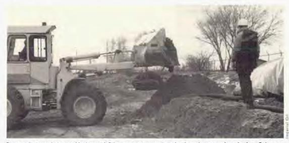
Bioremediation is being used by Imperial Oil to restore contaminated soils at their waterfront lands in Cobourg. The natural bacterial process that degrades hydrocarbons in the soil is enhanced by creating piles of soil and adding nutrients and oxygen.
